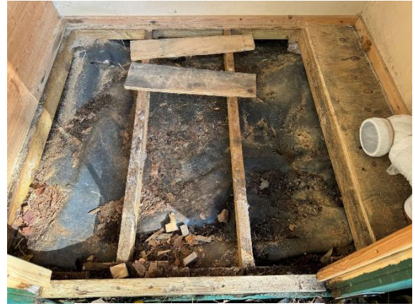
Uncovered, a bit of a mess.
