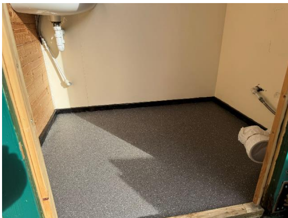
New vinyl floor covering laid and walls painted
