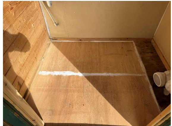
New boards fitted and sealed up
