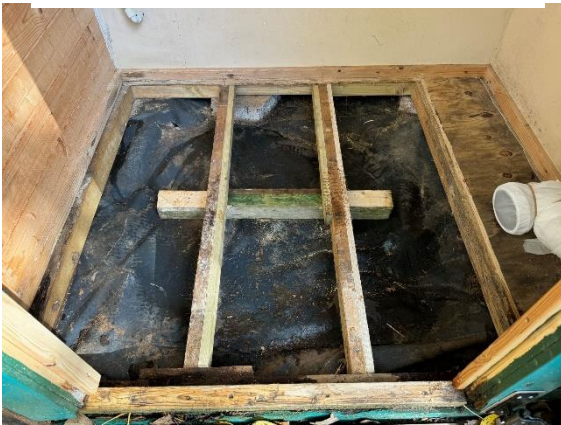
Floor joists strengthened and supported
